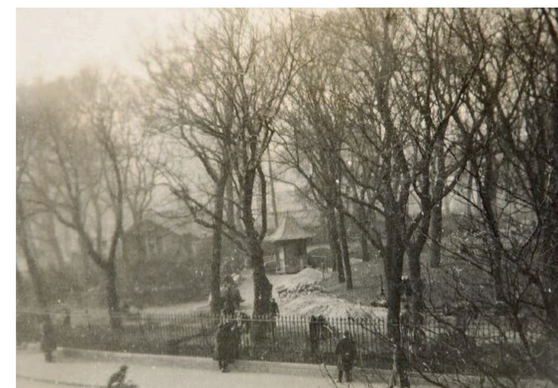
Removal of railings 1923
